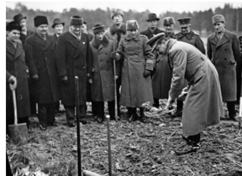
22.12.1938 Marshal Mannerheim dug the first shovel to start the construction of the Olympic Indoor Arena in Helsinki
